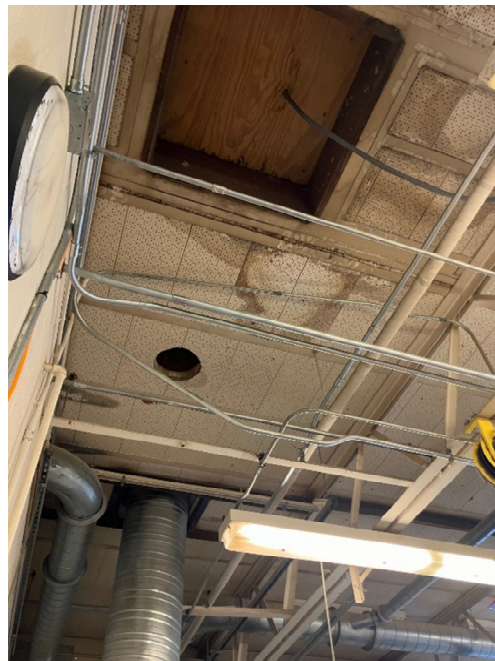
HS Roof 9 – TL-2
