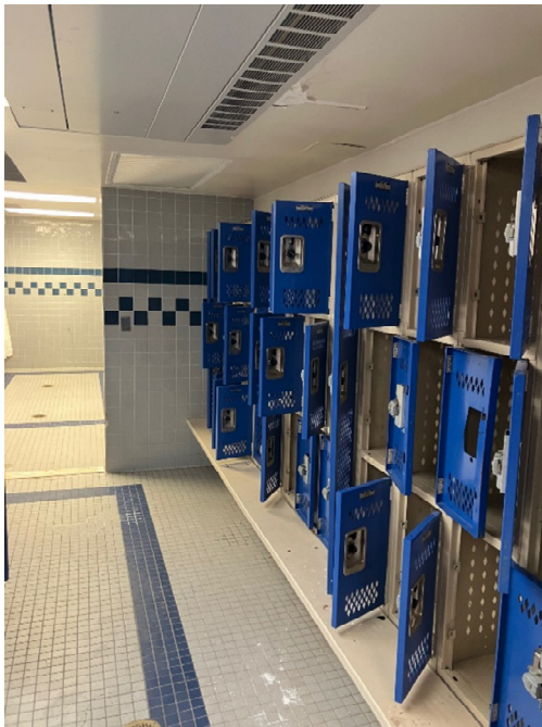
HS Roof 13 – Boys Locker room
